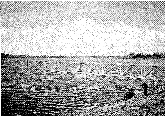
Water Reservoir KM35 (Savannakhet)
