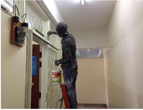
Applying “Anti-MosQ” paint
